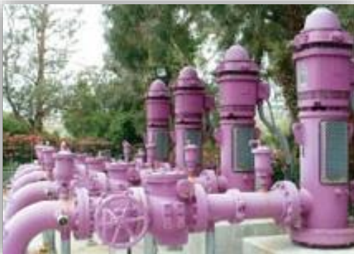
Photo by: Metropolitan Water District of Southern California.
