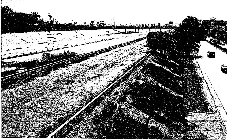
TIJUANA RIVER FLOOD CONTROL CHANNEL PHOTO 1
