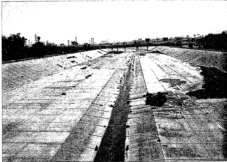
TIJUANA RIVER FLOOD CONTROL CHANNEL PHOTO 2
