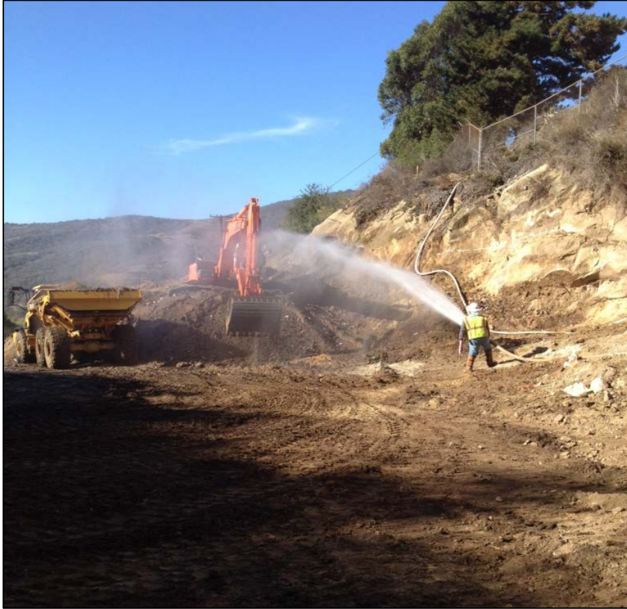
Water Tank Ravine Burn Site, Primary Area excavation and dust control
