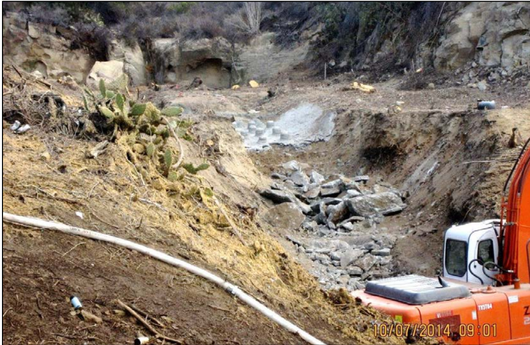
Water Tank Ravine Burn Site during Waste Removal
