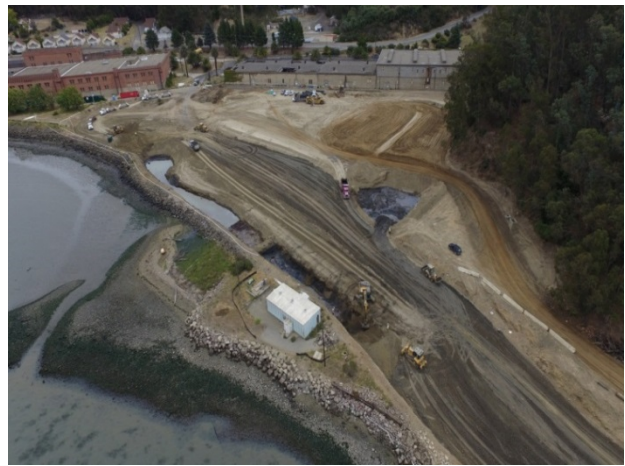
Photo 3. Aerial image of IR Site 3 during excavation.
