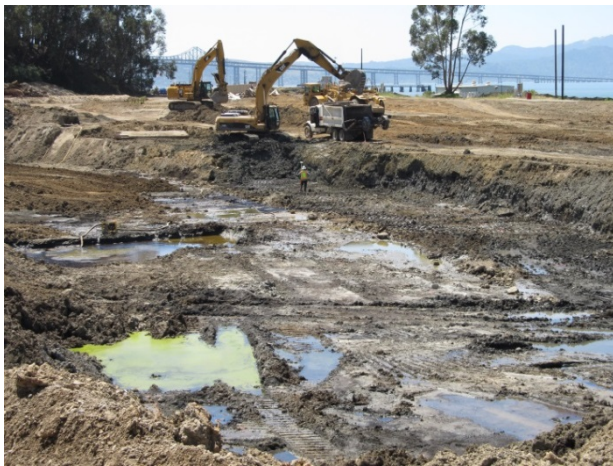
Photo 2. IR Site 3 during excavation.
