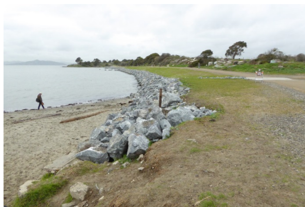
Photo 2. Landfill shoreline after construction.
