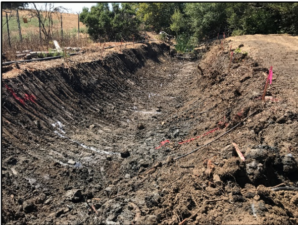
Figure 3. Excavation of IR-8 Drainage Channel
