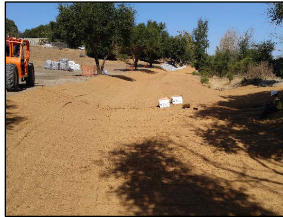
Figure 4. Completed Drainage Channel with erosion control matting
