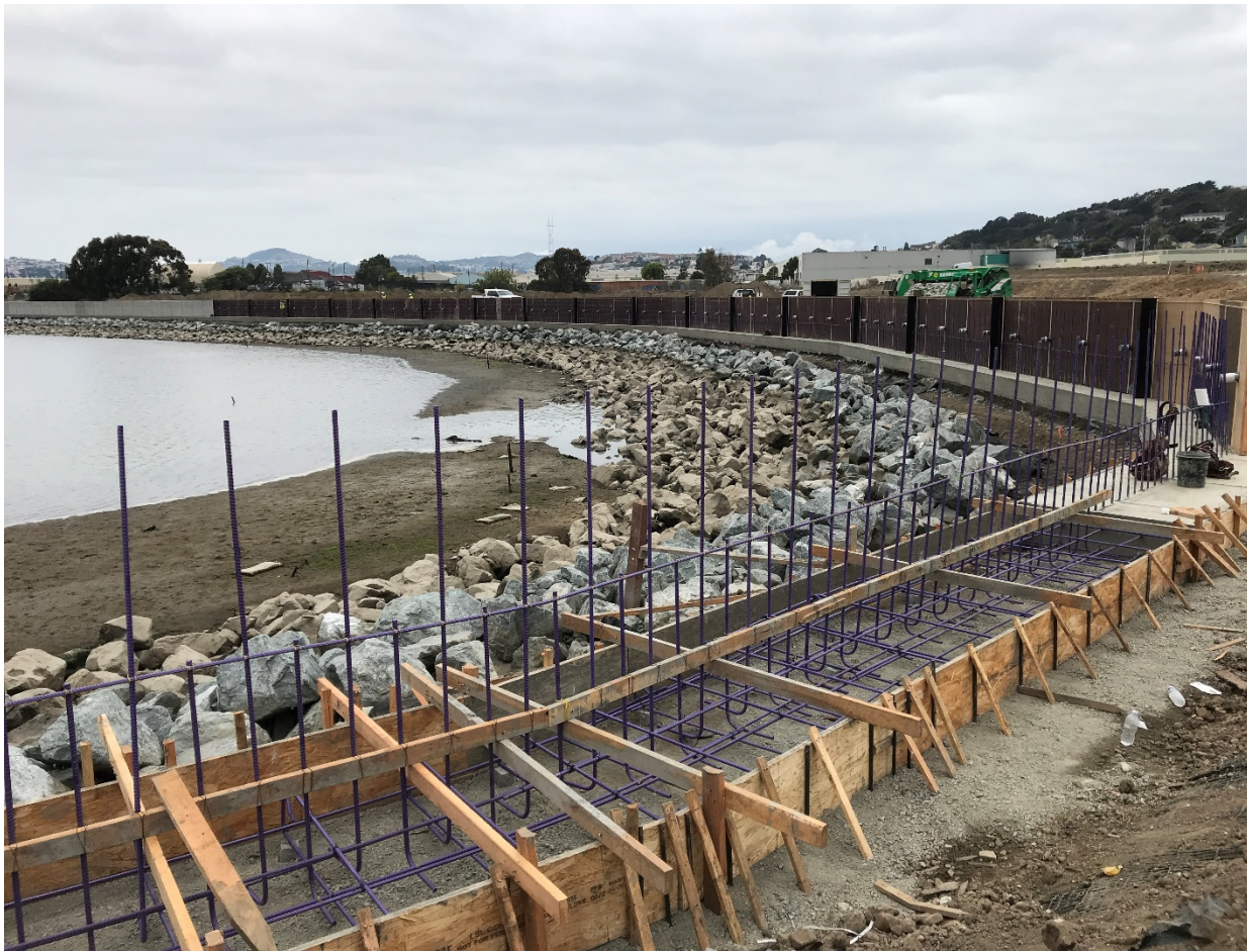
Figure 2. Construction of the parcel E-2 seawall and revetment (August 30, 2018)
