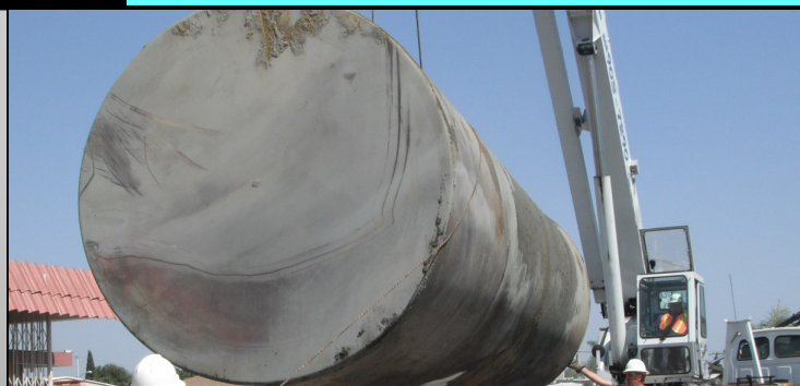
Photo: Removal of a UST at a former gas station
