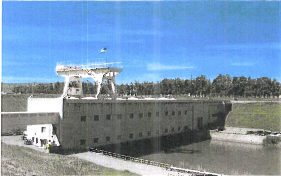
(5) Central Valley Project – C.W. "Bill" Jones Pumping Plant
