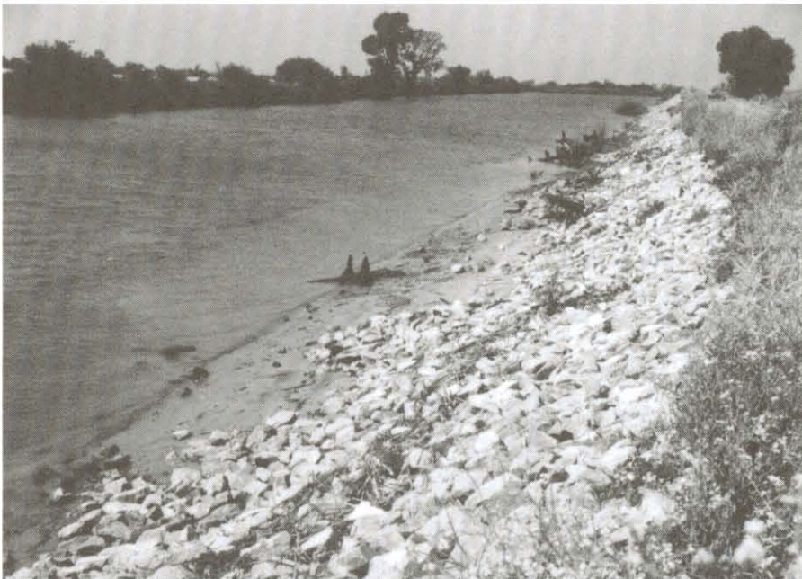
Some levees are protected from erosion by riprap.
