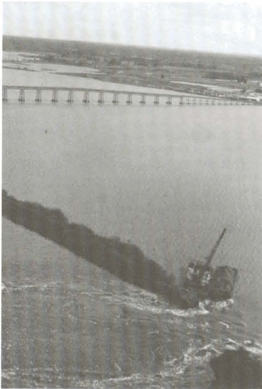
Levee break on Sherman Island in 1969.
