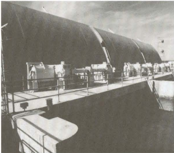
The Suisun Marsh Salinity Control Gates began operating in 1989. Each of the three gates measures 36 feet wide by 28 feet high and operates electronically to improve water quality in the marsh.
