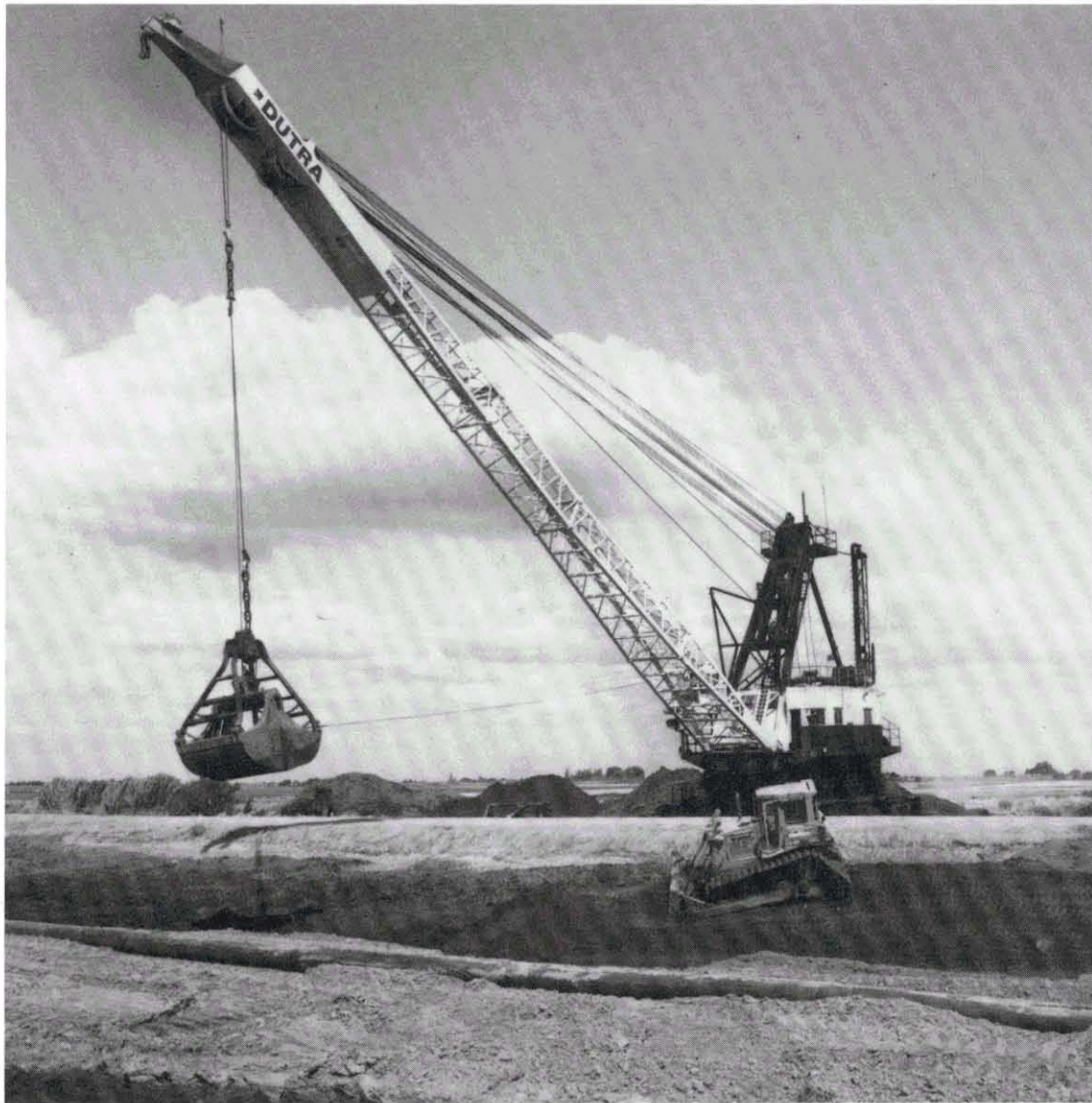
Levee rehabilitation on Twitchell Island.
