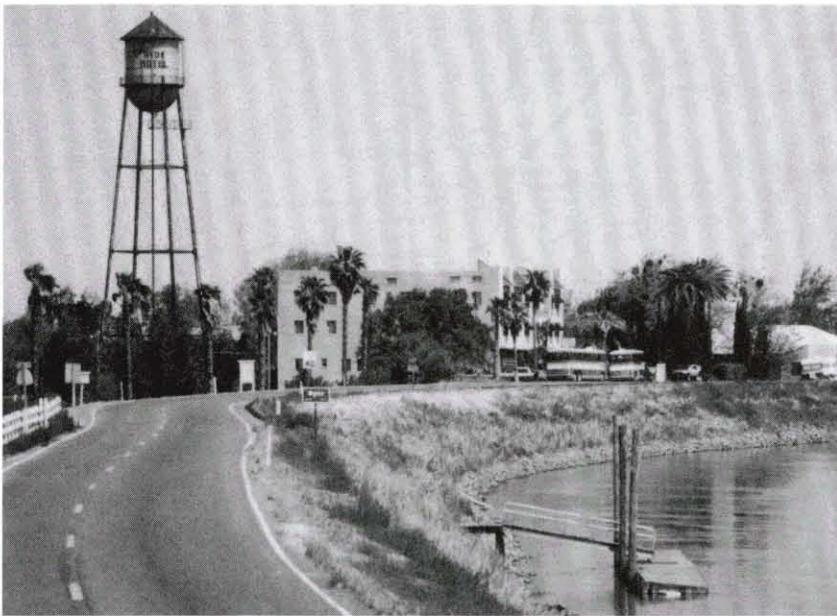
The town of Ryde is one of many communities protected from flooding by project levees.
