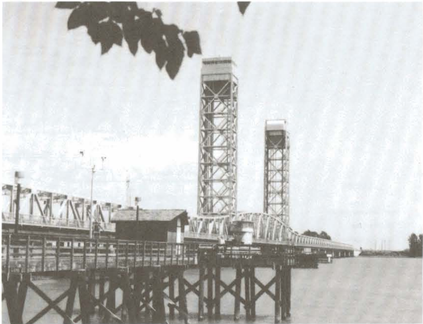
Rio Vista bridge on State Highway 12.
