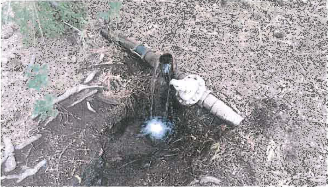
Discharge of water diverted at Pre-1914 well. Pipe disconnected from distribution system (at right).
