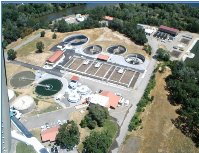
Clear Creek Wastewater Treatment Plant, Redding CA, photograph courtesy of Central Valley Regional Water Quality Control Board
