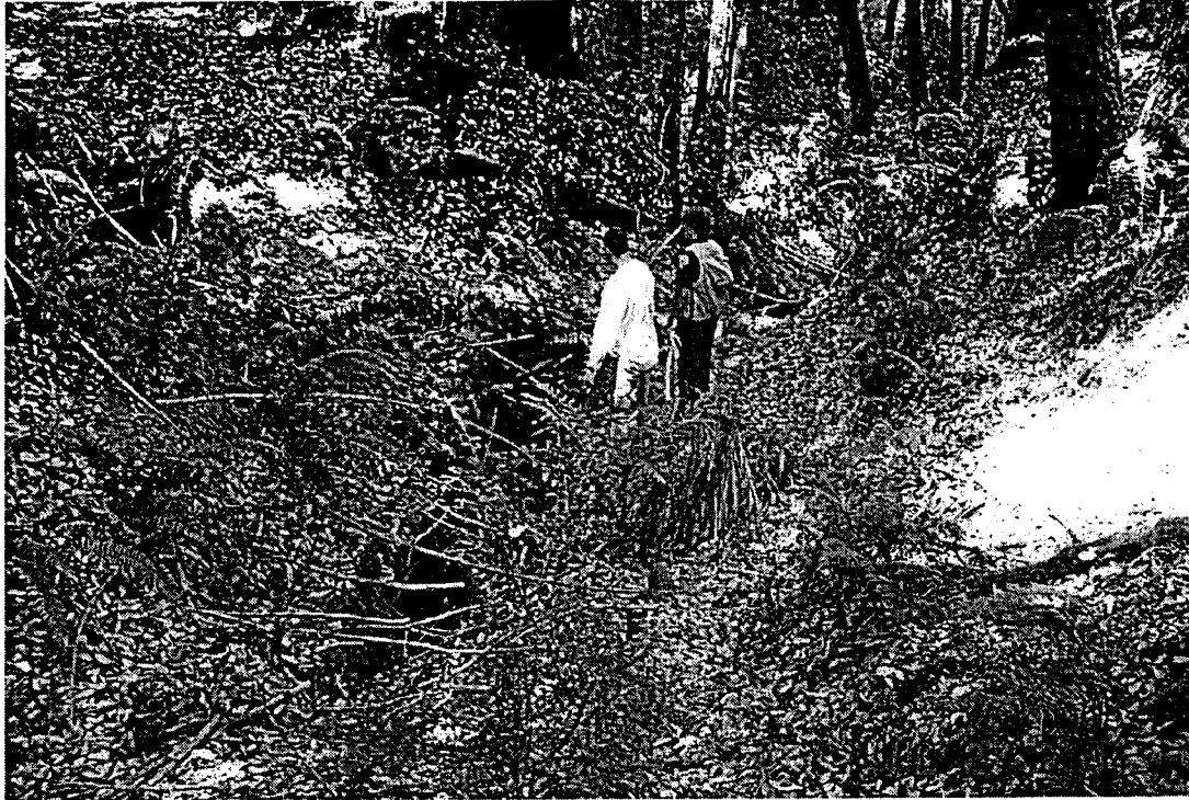
Figure 4. Mr. Fitzgerald and Ms. Petersen inspecting the lower part of the Class II watercourse, where the channel is considerably more incised.
