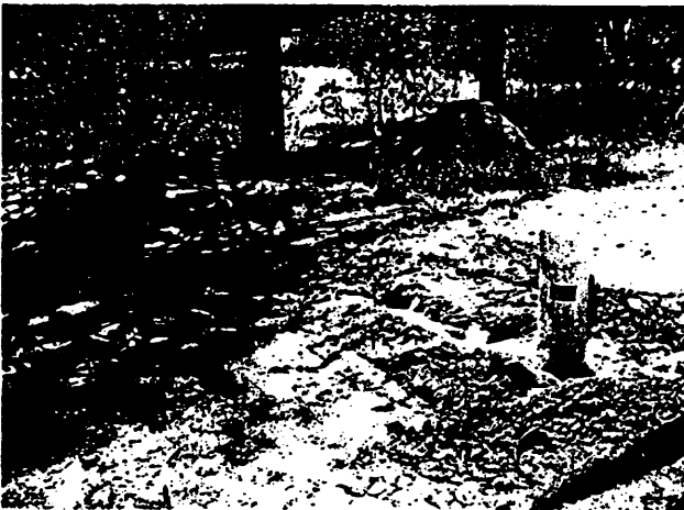
Photo 1 - Drill mud and bentonite around wellhead
