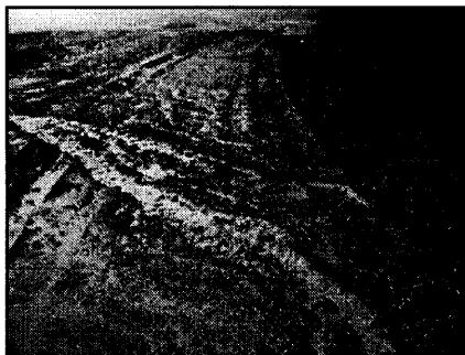
Below and Right: Greens Complex 1 area with no erosion control, unprotected stock piles, and failing sediment control. Discharge of sediment-laden water to surface waters.
