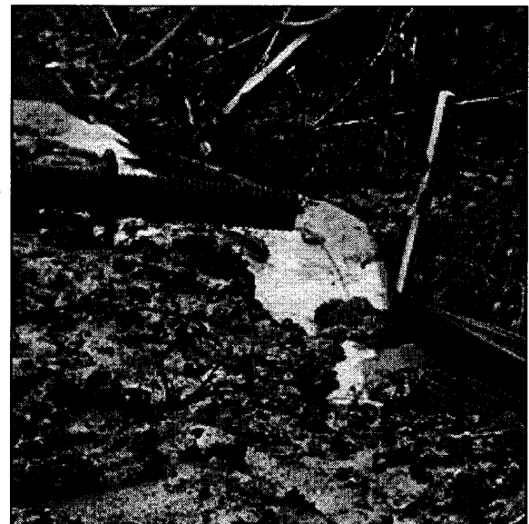
Above: Erosion at Greens Complex 18 and storm water drainage into pipe. No erosion controls.
