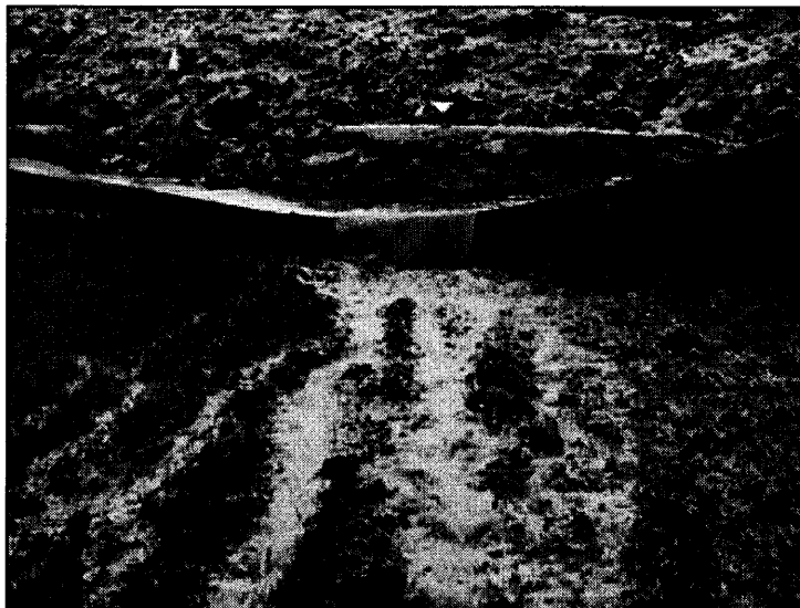
This Page: Sediment overwhelming silt fences in Greens Complex 5 area. Widespread erosion and no erosion controls in disturbed areas. Discharges of sediment to surface waters.
