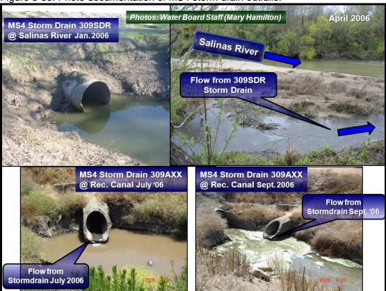
Figure 3-39. Photo documentation of MS4 storm drain outfalls.
