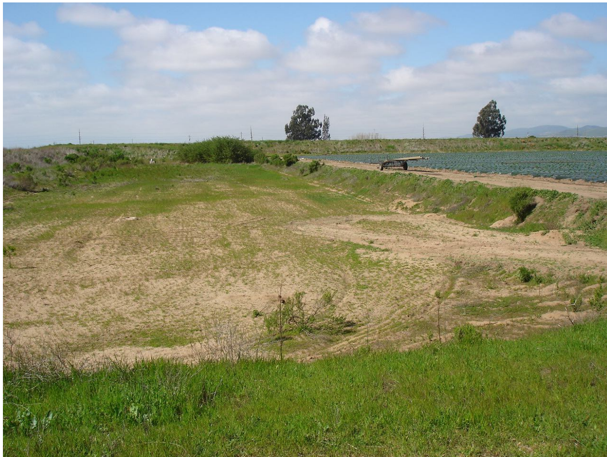
Figure 15. Sediment basin at the edge of farm field in the Salinas River watershed
