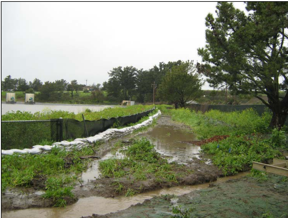
Impoundment facility flooding – February 17, 2017
