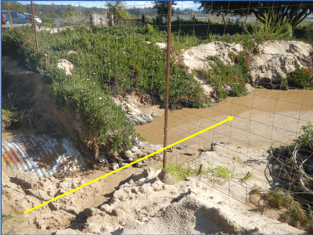
Discharge from culvert to unmaintained sediment basin
