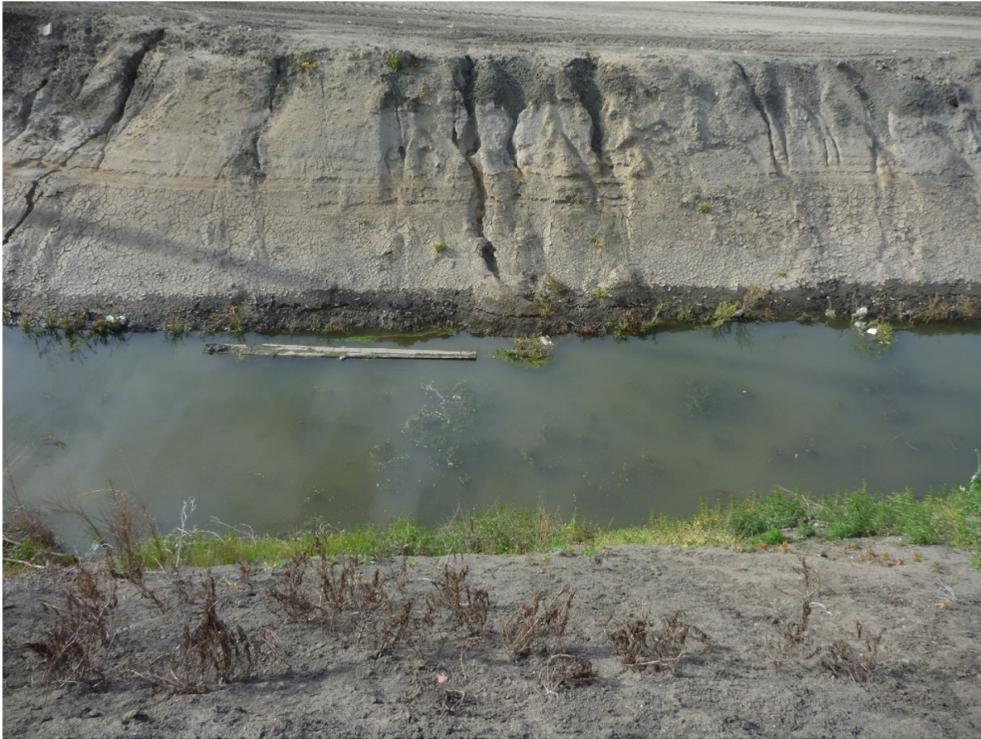
Figure 28. Photo of bank rilling and erosion the Salinas Reclamation Canal upstream of Highway 101. Source (MCWRA, 2015a).
