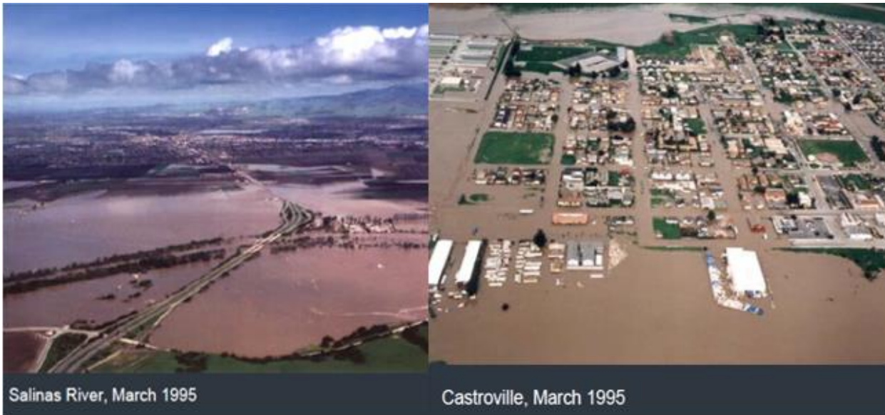
Figure 10. Photos taken from the air of flooding in the lower Salinas River watershed after a large storm event, March 1995 (MCWRA, 2015).
