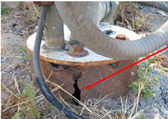
A cracked well casing may allow surface water and contaminants into your well. One of the most common water quality issues associated with a cracked well casing is the presence of coliform bacteria. Other chemicals can also be introduced into the well through the cracked casing. Consult a water quality professional, like a licensed well driller to repair or replace the cracked casing.
