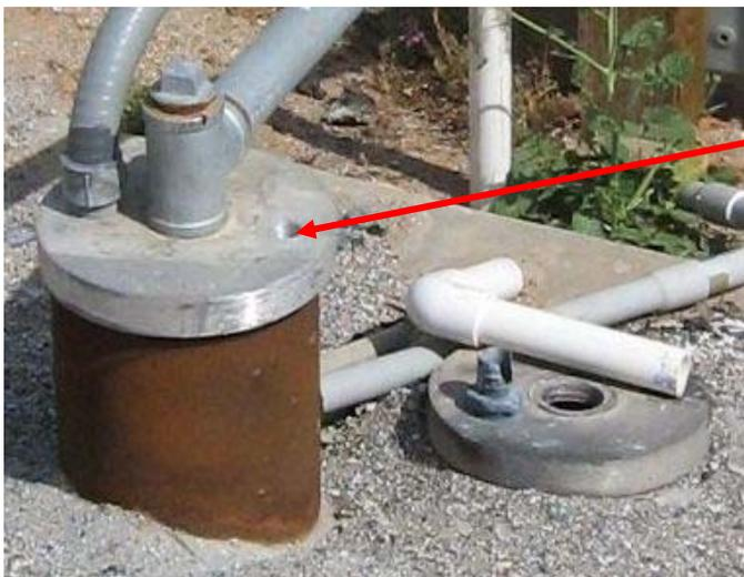
Many wells have a small plug located at the top of the well casing. The plug may degrade over time and sometimes fall off. If the plug is missing, the well is directly open to potential contamination. The most frequently observed contaminant associated with a missing plug are coliform bacteria. Replacing a missing plug is an effective way to reduce potential contamination.
