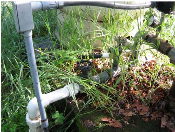
Overgrowth of vegetation near your well may lead to root damage of the casing, creating a conduit for possible well water contamination.
