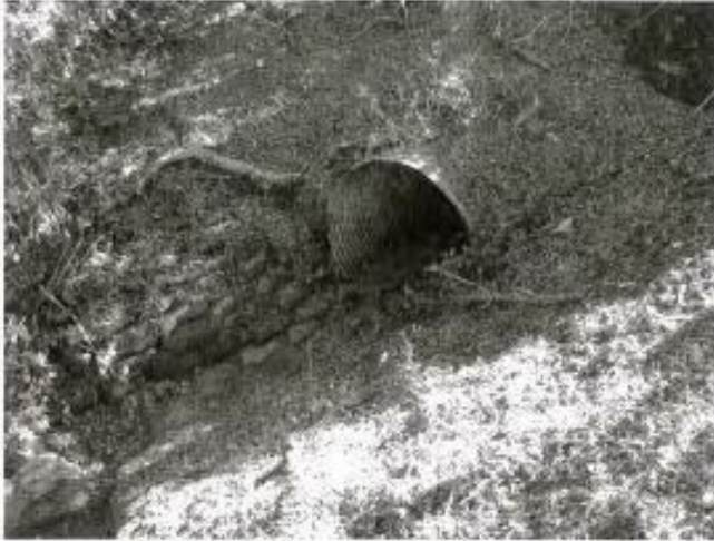
Culvert outlet showing SCSP.
