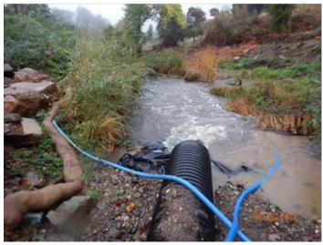
Photo 2. Clean water discharging downstream of the bridge project. Note: blue hoses used to dewater the construction area.
