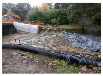
Photo 8. View of diversion dam as water was starting to overtop north end.
