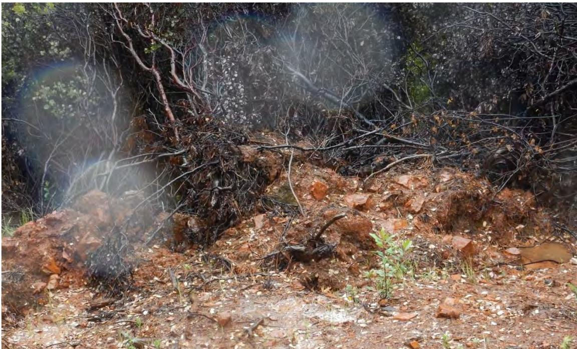
Photo 56: Unprotected cut-slope from bottom terrace to second terrace.
