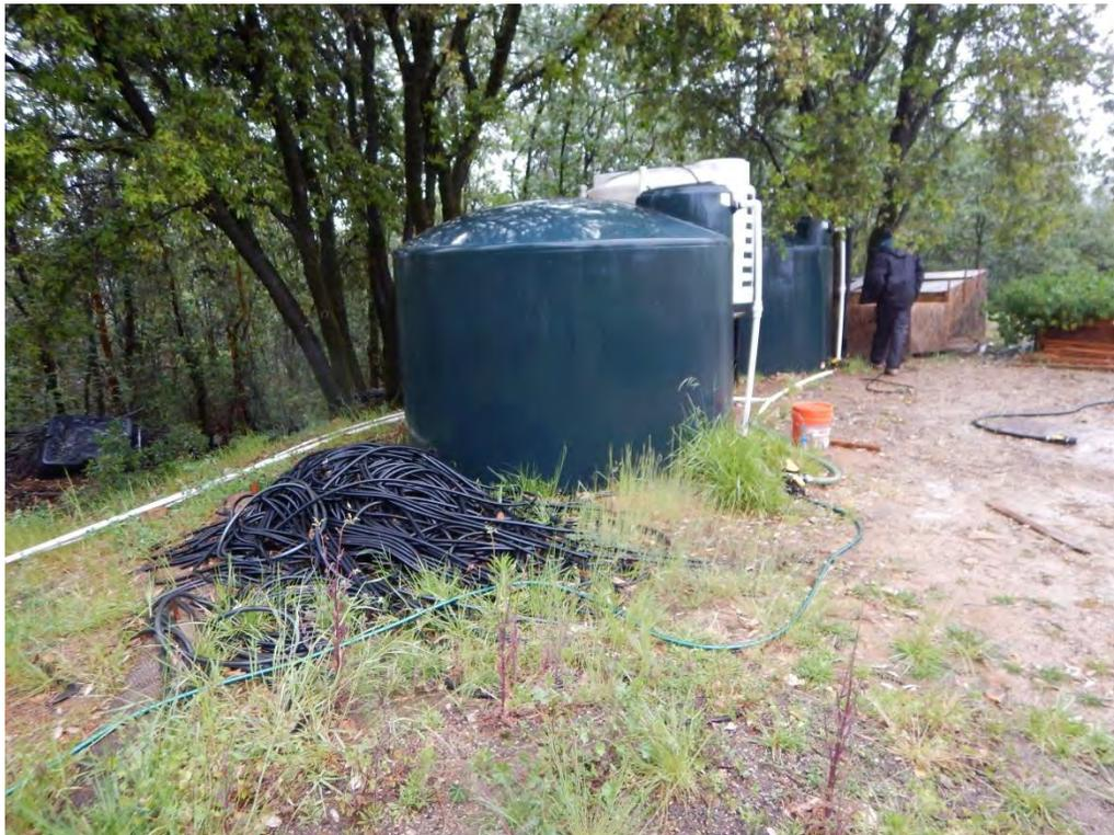
Photo 26: Irrigation pipes from the storage tanks. Weathered staked straw waddles installed behind the water tanks—providing little protection from runoff and erosion.
