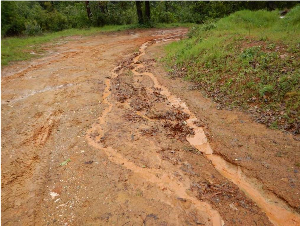
Photo 7. 6-8 inch deep rills formed from storm water runoff and erosion of clay soils.
