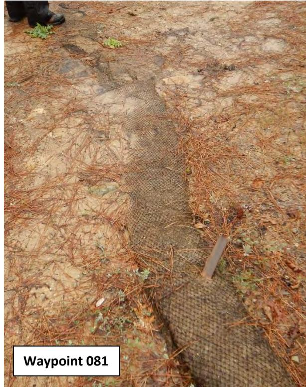
Photo 51: Terrace Access Road on western end of properties showing channelization and rilling.
