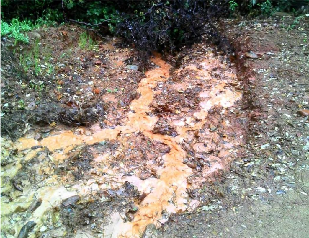
Photo 12. Turbid sheet flow exiting road into forested drainage through ineffective slash. Way Point 087.
