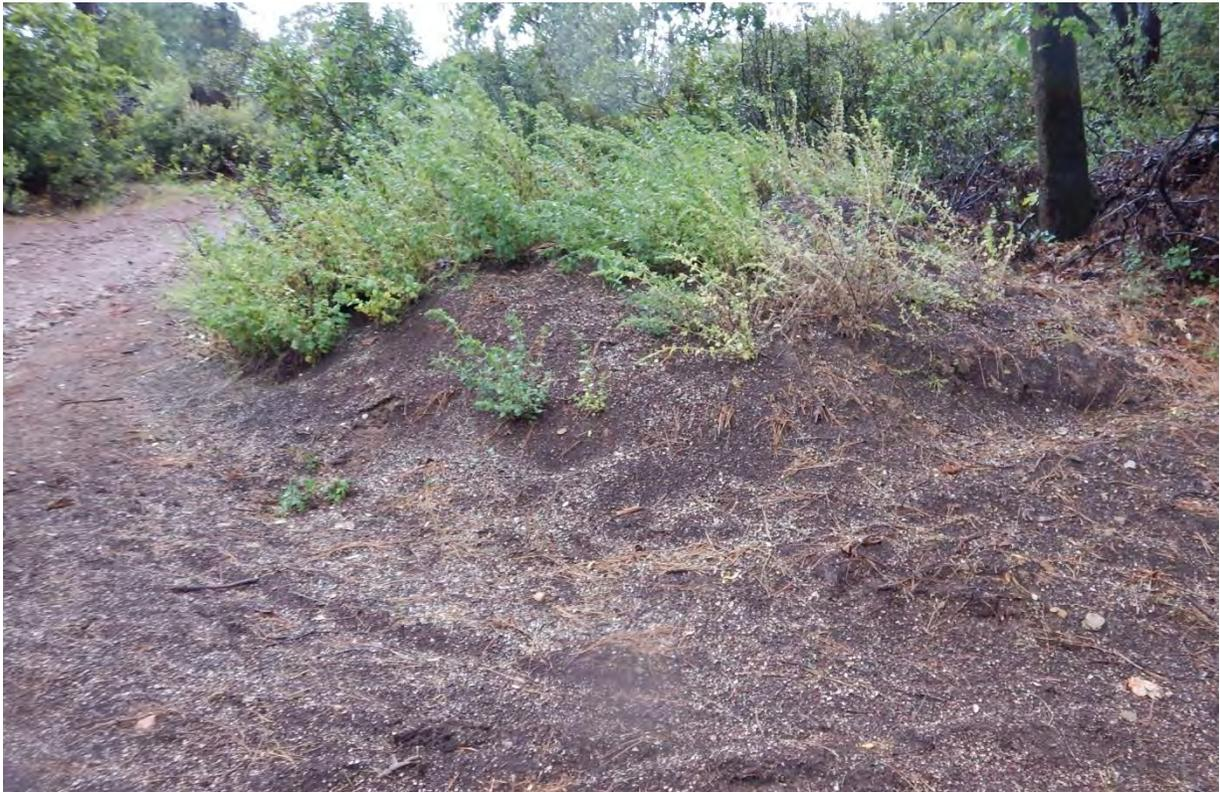
Photo 35: Additional potting soil contained by straw waddles.
