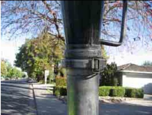
3e. Pipe secured to cone with clamp.
