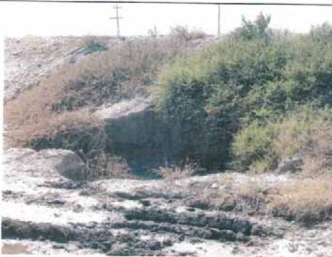
**Photo 2:** Large hole on the eastern embankment of the 'Big Reservoir.' It appeared to staff this hole compromises berm integrity.
