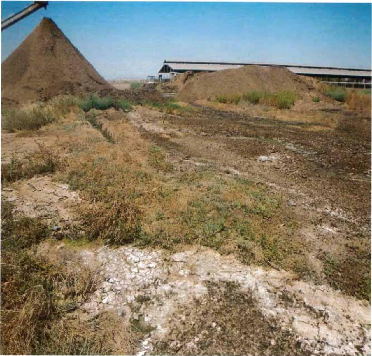
Photo 1: Photo of the uncontained manure stacking area without proper drainage.
