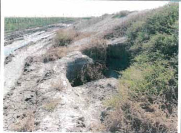
**Photo 3:** Large hole on the eastern embankment of the 'Big Reservoir.'
