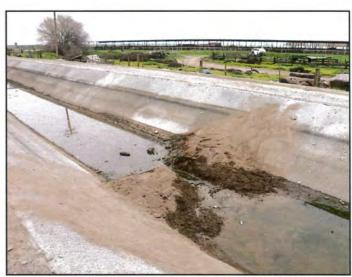
**01 22 2015** – View southeast showing berm in MID canal; note breach in center of berm.
