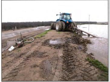
View east down north berm of Lagoon 2 showing pump intake at right and point of discharge at left; note lack of freeboard.
