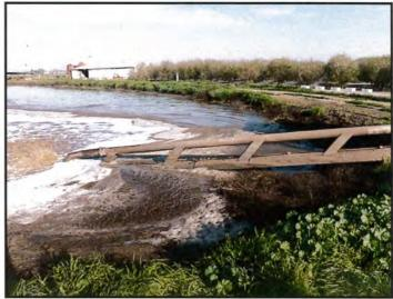
**02 26 2015** – View northwest across east end of Lagoon #1; note lack of freeboard. The pipe is part of the pumping mechanism for applying wastewater to cropland.
