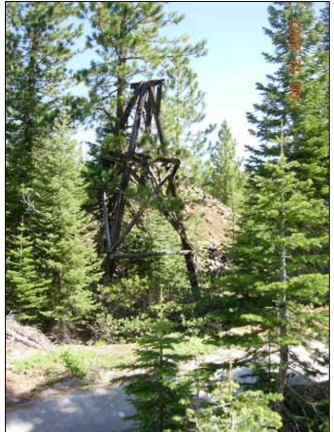
22. Photo of a tower structure for the former aerial tramway that moved supplies and materials between the Walker Mine and Quincy. Shotcrete-lined diversion ditch in the foreground.
