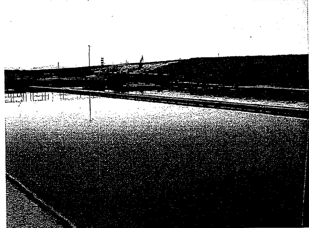
Photograph 4. – View of the wastewater sumps looking southeast.
