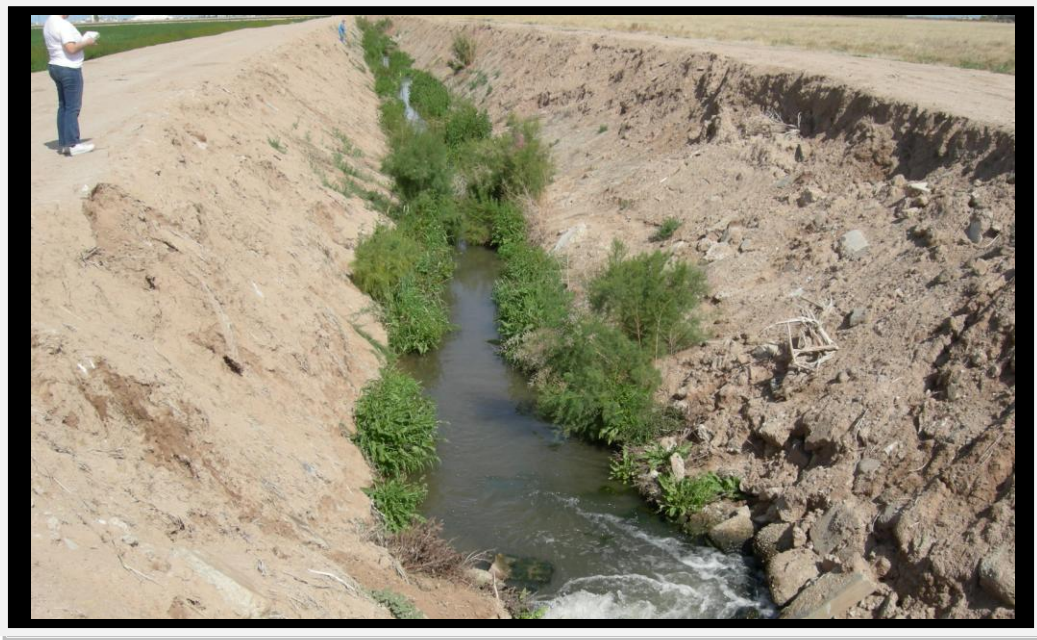
1. Dolson Drain at Wastewater Pipe Discharge 32°51'17.5"/115°33'10.6" (WGS 84 EPE 17 feet)
