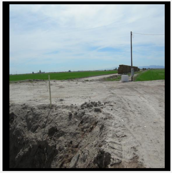
2. Field Pump to South of Start of Dolson Drain
