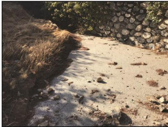
**Photo 4:** View illustrating the transition from Drainage 1 (soil and annual grasses) to Ditch 1 (cement-lined channel).
