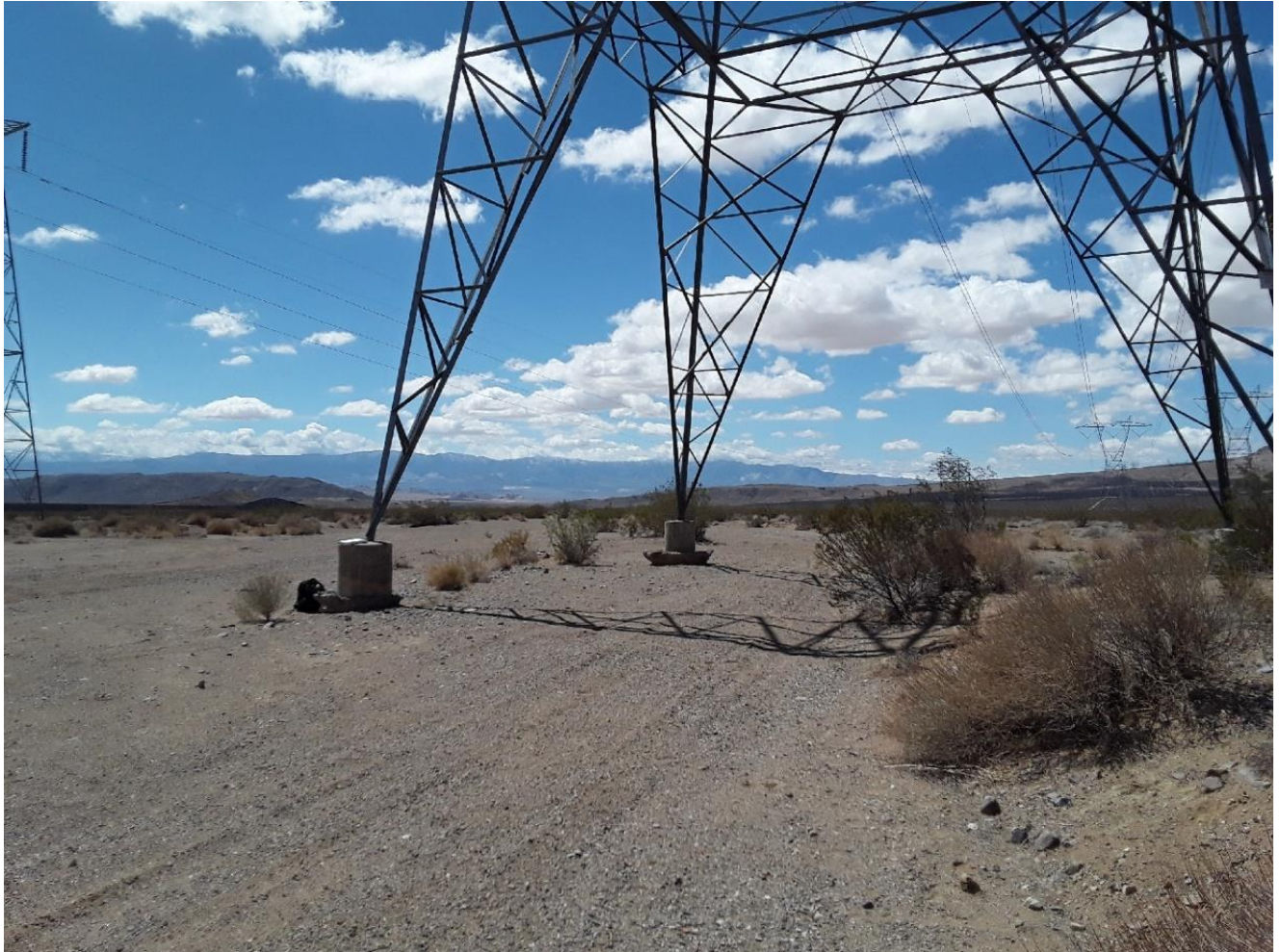
Photo 2: M42-T2 tower base footings in wash. Photo facing southwest, downstream.
