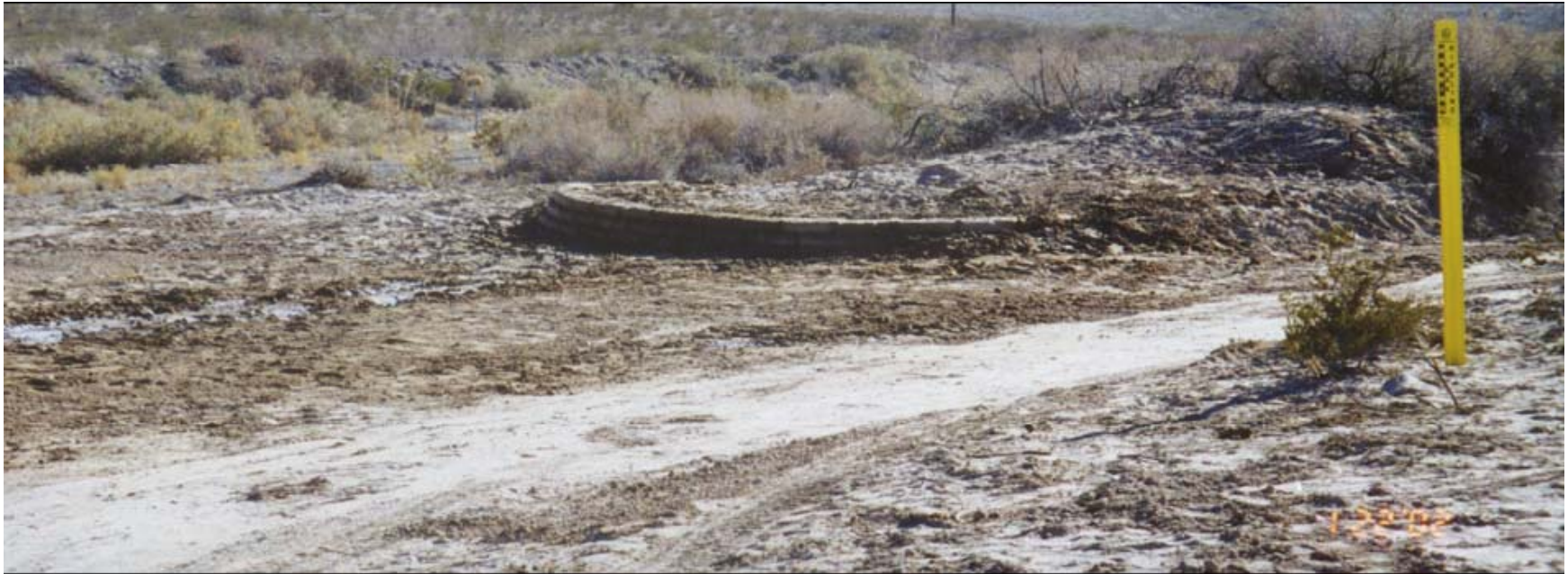
Photo 3: Example of an existing FCR structure in an ephemeral channel of California. (photograph courtesy of Ercon)
