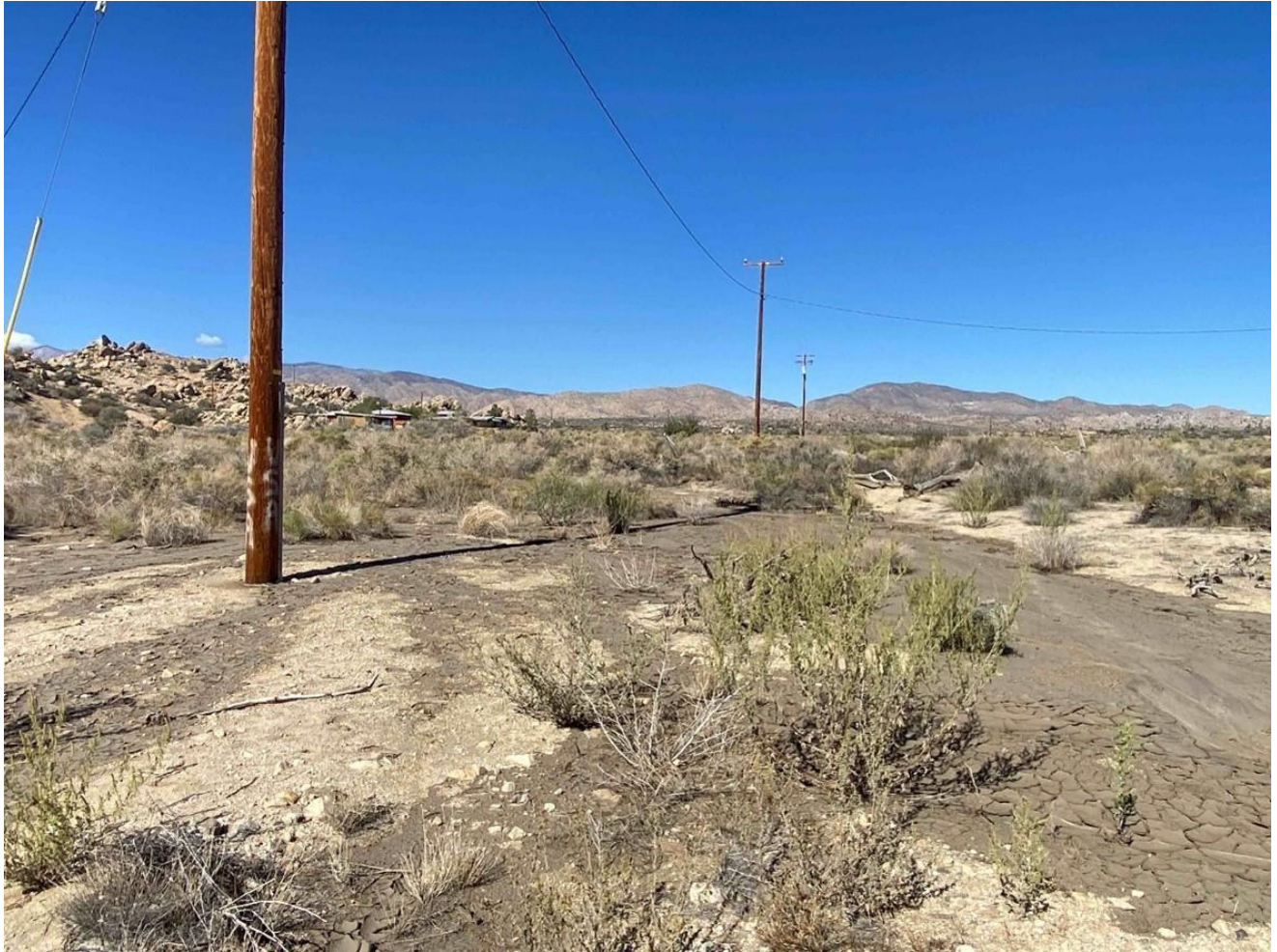
Photograph 1. Pole 4665313E overview. Photo taken facing northwest west (upstream).
