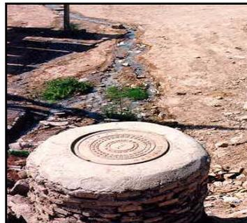
Figure 91: Overflowing sewer manhole (Apr 1988)
