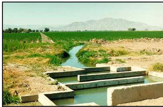
Figure 81: Distribution system for effluent irrigation from Mexicali sewage treatment lagoons (Mar 1987)
