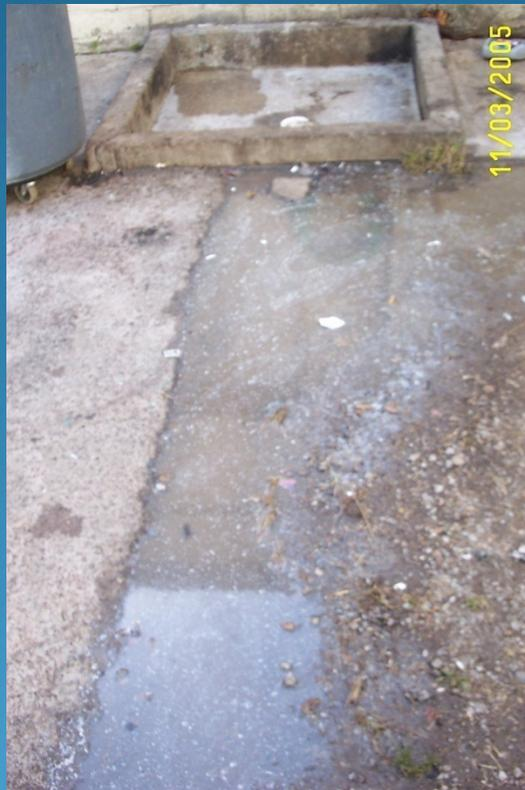
Uncovered Mop Sinks cause I/I to sewer system and many times the mop sinks are upstream of the grease interceptor. Outdoor mop sinks should be covered.
