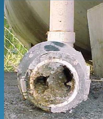
Outlet pipe of trap with no flow restrictor
