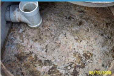
Proper schedule 40 PVC Inlet T  $\frac{1}{2}$  to  $\frac{2}{3}$  the depth of the tank (picture at right) prevents back-ups into FSE, and does not allow the influent wastewater to push the FOG layer down and allow shortcircuiting.
