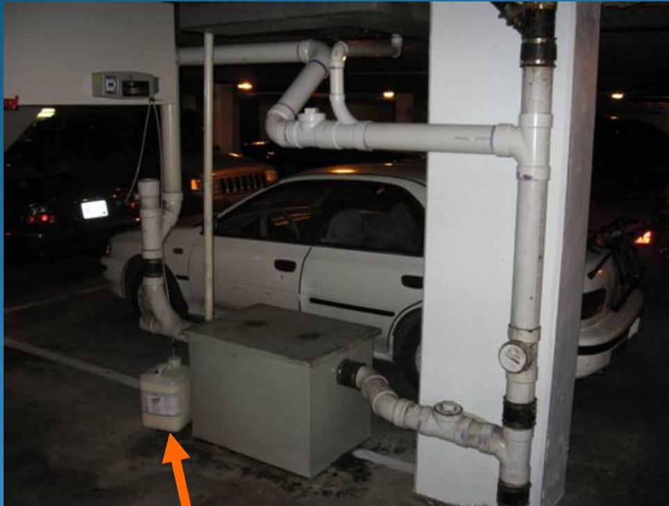
Trap in basement with additives (enzymes) added before trap. Heavy FOG in downstream sewer line.
