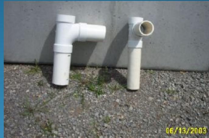
Outlet Ts can be too short, allowing shortcircuiting. Some rely on baffle in front of outlet pipe but this is not efficient for FOG control
