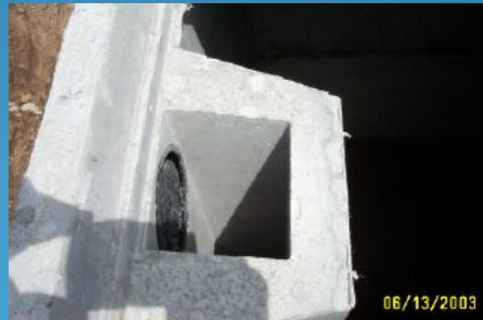
Flexible outlet Ts attached to wall: NOT ACCEPTABLE
