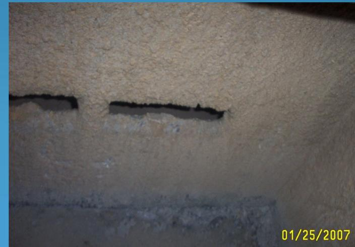
Mid-wall Baffle (or 2/3 baffle wall)- deterioration. Will probably need interceptor certification to confirm deterioration or leaks (gravel in bottom of tank in many cases is indicator)
