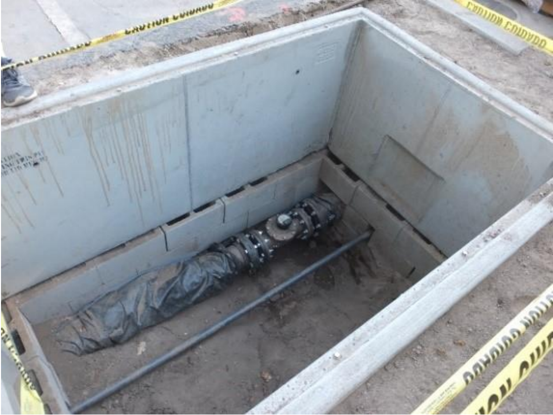
Photo 2 New meter installed into system
