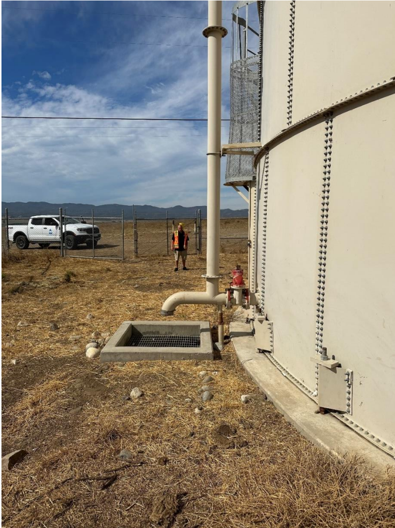
Overflow Drain and Piping
