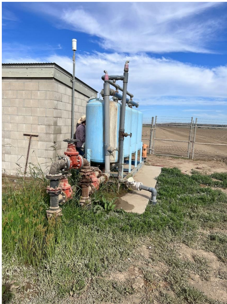
Manganese Dioxide Filtration System
