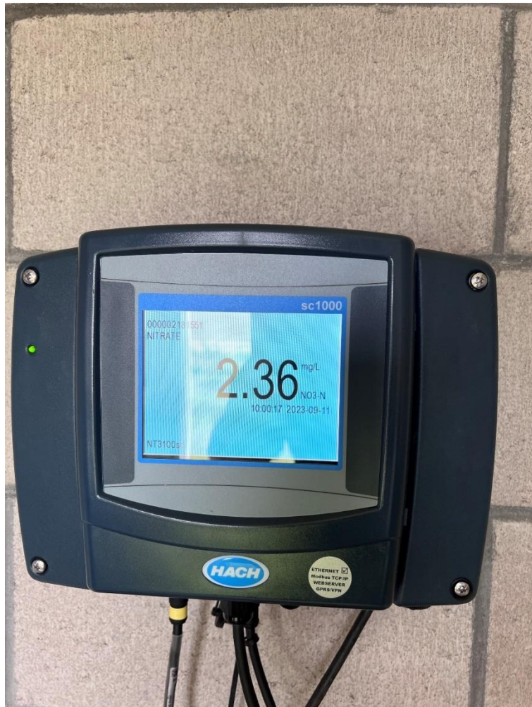
Multi-Parameter Online Analyzer Display
