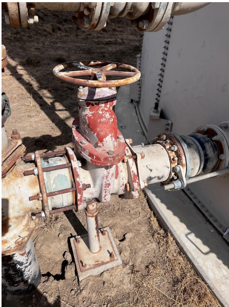
Outlet Flow Control Valve
