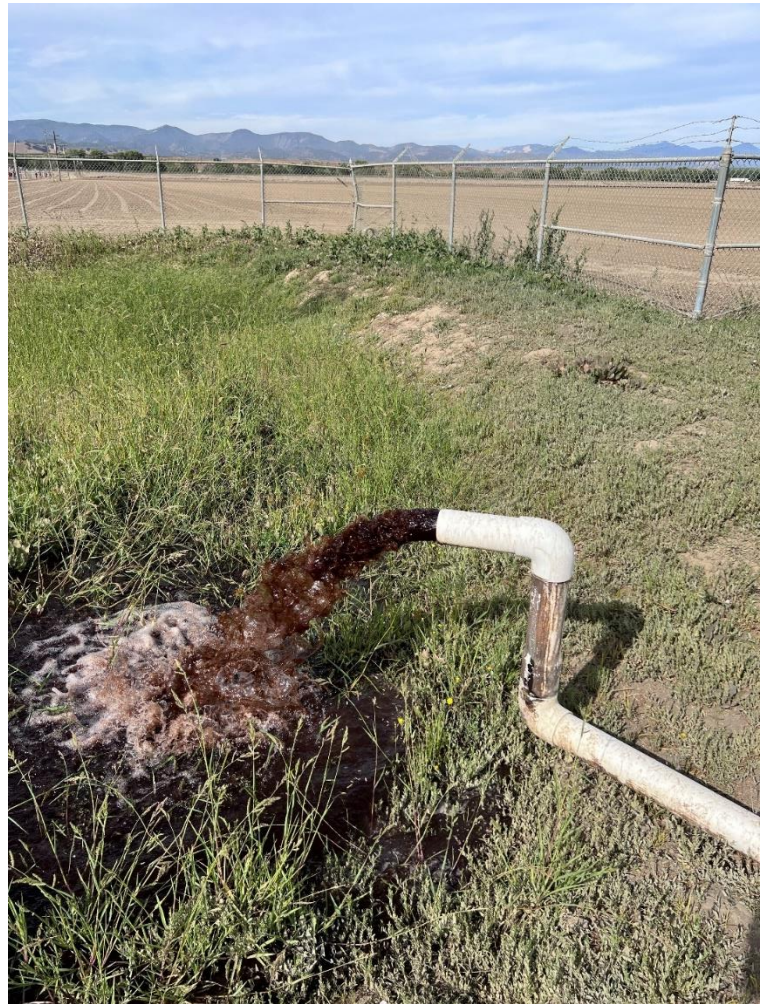
Wastewater from Filter Backwash
