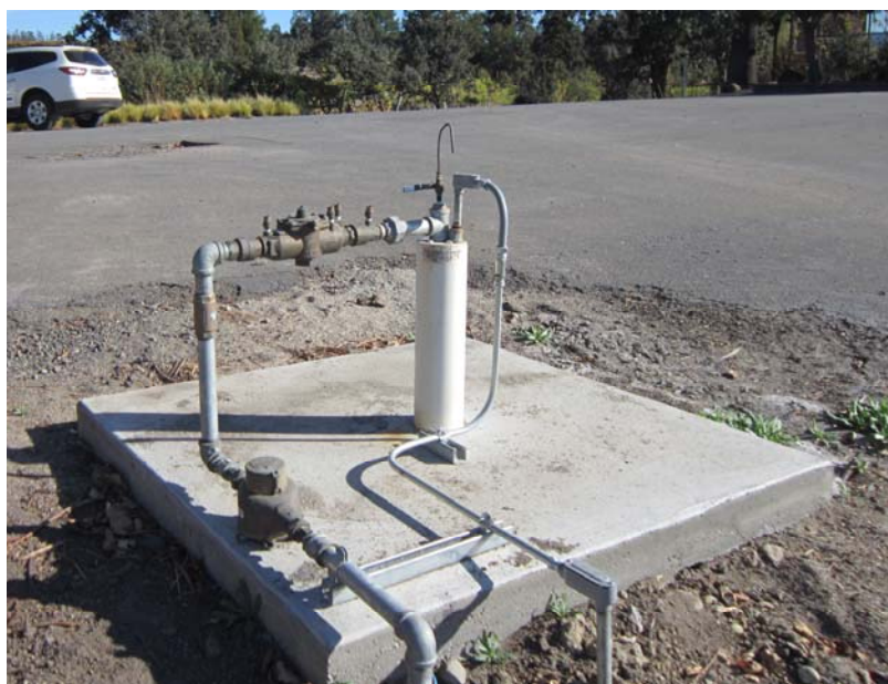
Properly constructed wellhead.
