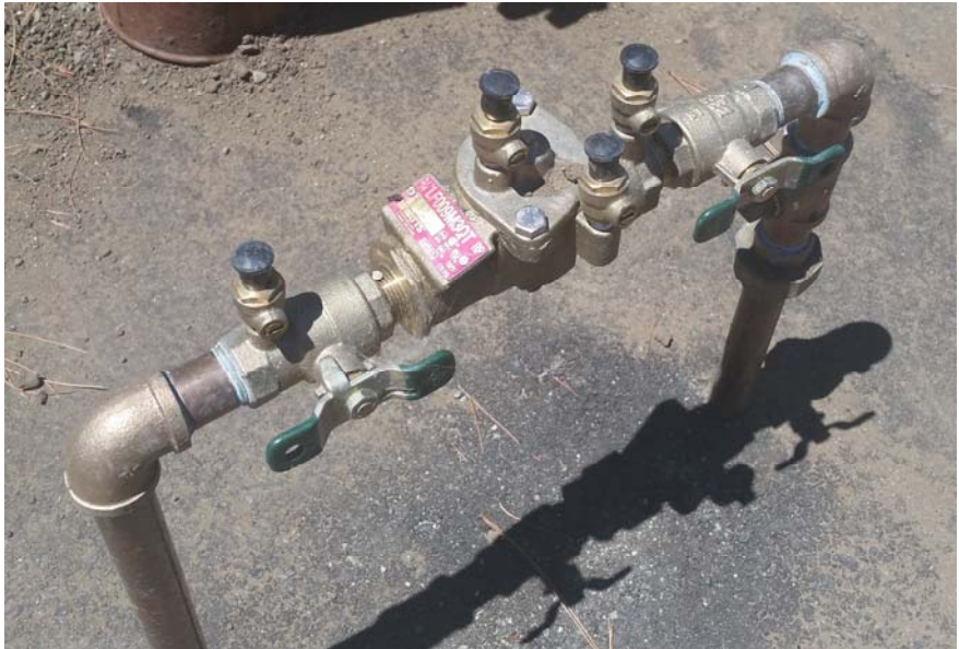
Reduced pressure assembly
