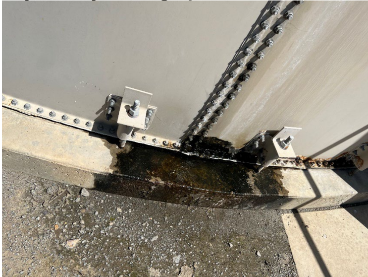
Leak 1: First observed in 2020 Sanitary Survey. Still present
