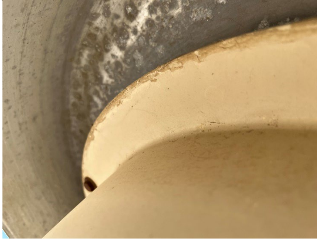
Storage Vent does not have a non-corrodible screen.
