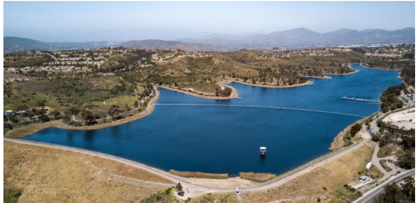
Figure 3-4: Miramar Reservoir in San Diego County showing the top of the intake tower
