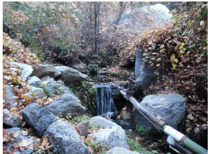
Figure 3-1: Chino Creek in Riverside County showing the surface water intake pipeline to the water treatment plant
