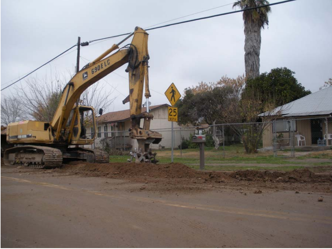
Water Main Installation
