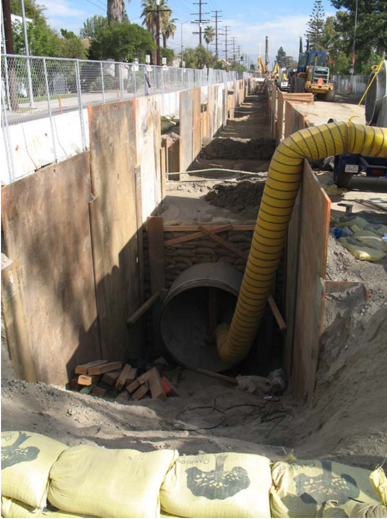
1910067-017 City of Los Angeles Project-Pipeline installation
