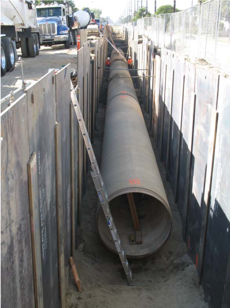
1910067-017 City of Los Angeles Project-Pipeline installation
