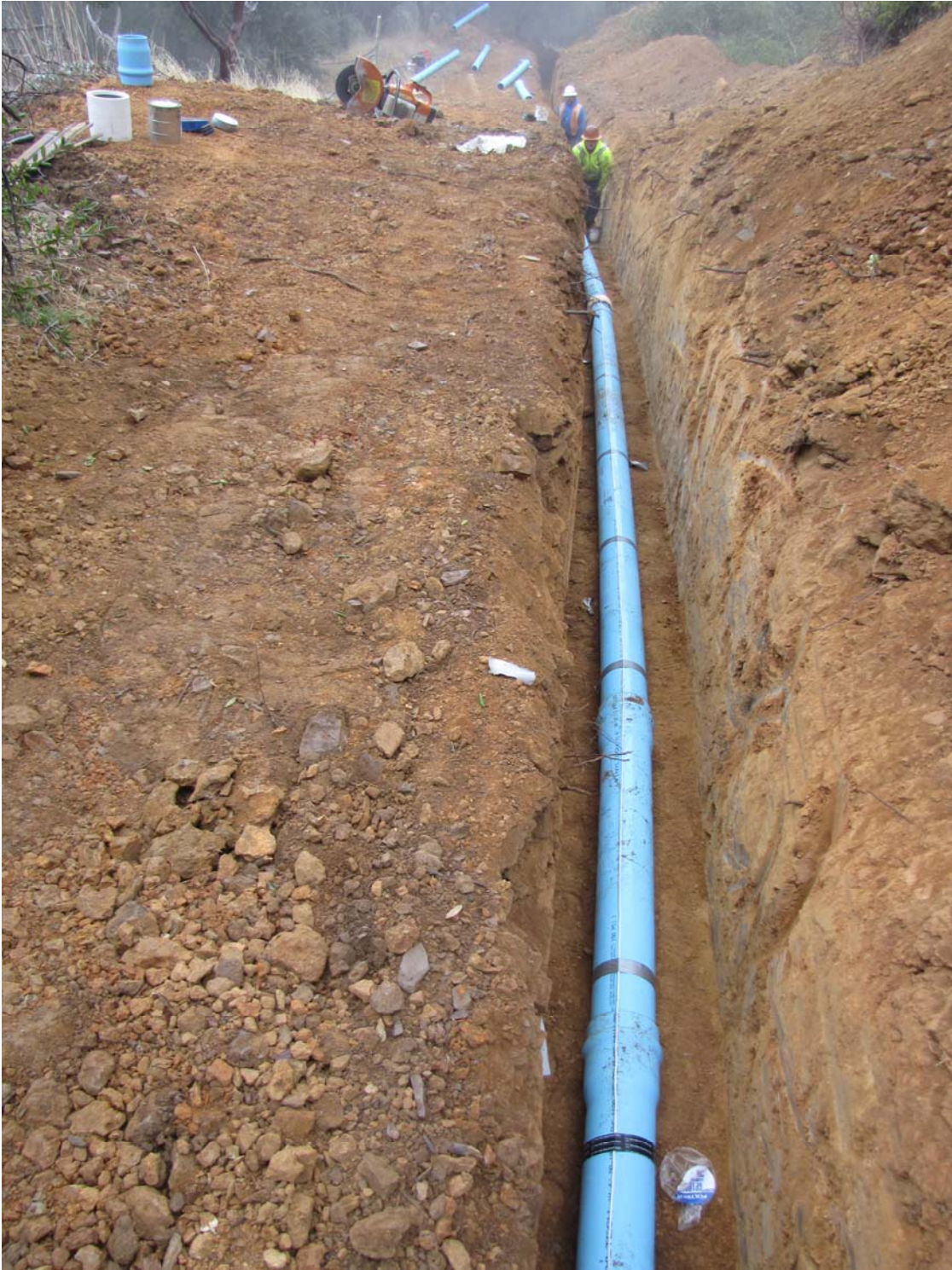
3700909-002 Julian CSD Project-Pipeline installation
