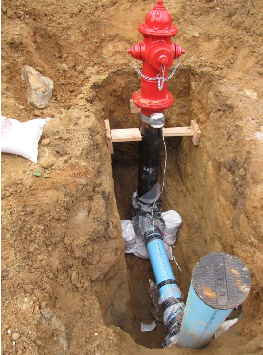
3700909-002 Julian CSD Project-Fire hydrant installation
