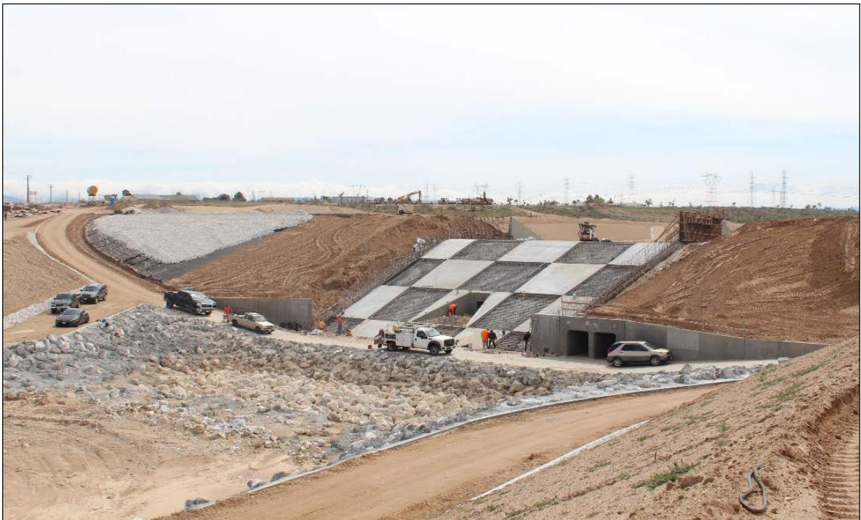
Figure 11b - View of the spillway still under construction and the two gated drain culverts
