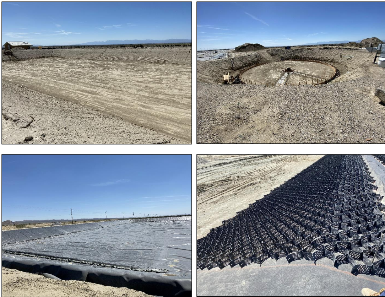
Figure 6.1 – Rosamond Water Reclamation Plant, May 13, 2020. Top Left: Excavation area of Biolac® aeration pond. Top Right: Excavation area for circular secondary clarifier. Bottom Left: Liner installation of emergency storage pond. Bottom Right: Geoweb® geocell installation on percolation pond side-slopes.
