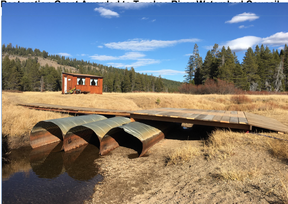
Figure 2.1. Failed culvert crossing, South Fork Prosser Creek. TRWC.
