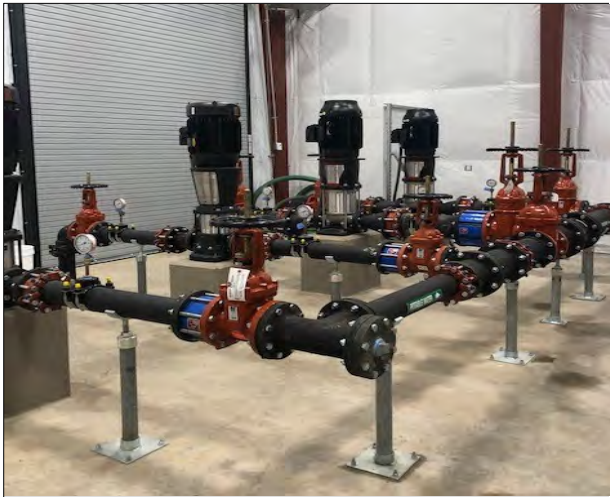
Figure 3.6: Booster pumps
