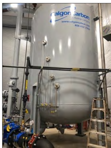
Figure 3.4: One of the two carbon vessels
