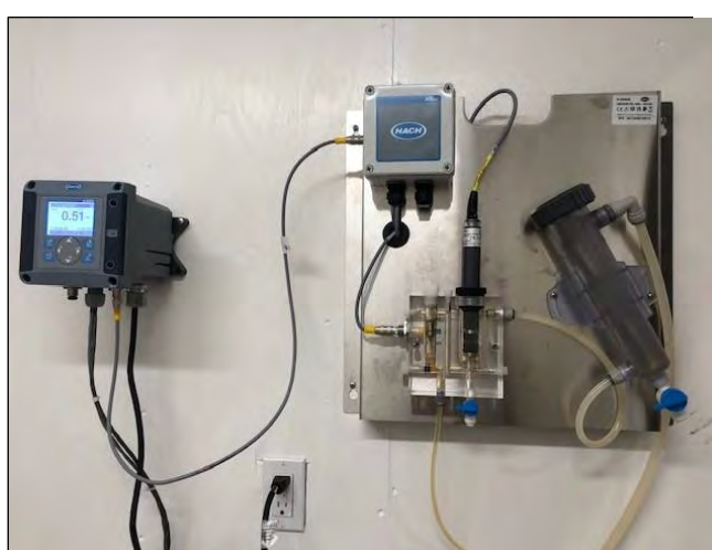
Figure 3.5: Chlorine disinfection system
